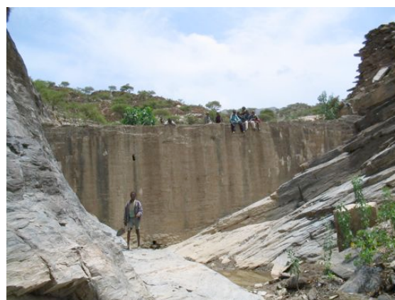
Illustration 14: Rebuilt cement check dam; T. L. 2002
