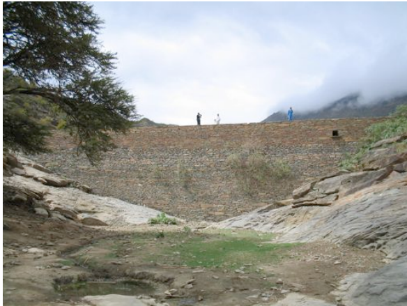
Illustration 29: Front view of the Alakalo check dam; July 2003
