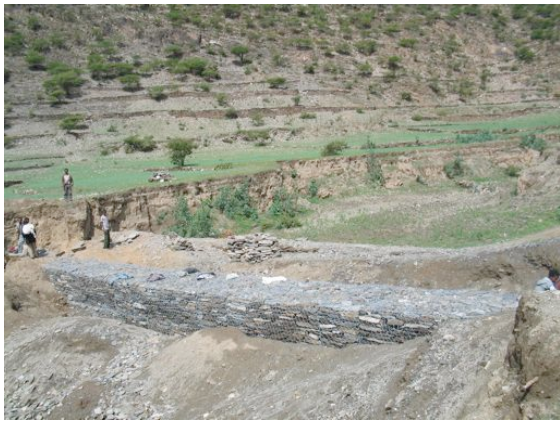
Illustration 38: Gully reclamation by a gabion check dam; August 2003
