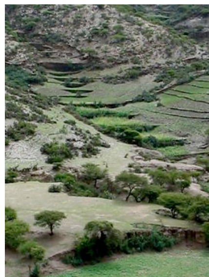
Illustration 2: Check dam sequence constructed by local farmers with cultivated maize fields in
