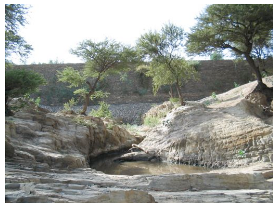
Illustration 10: Tikibta’s topmost check dam with part of its foundation; September 2003
