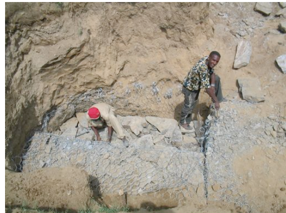
Illustration 39: Filling up the gabion with stones; August 2003
