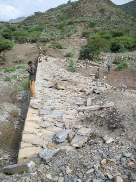
Illustration 36: Working on the check dam of Belguba in August 2003
