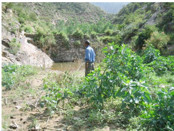
Illustration 27: 2 nd Intigade check dam field with obviously bad conditions for crop cultivating in September 2003
