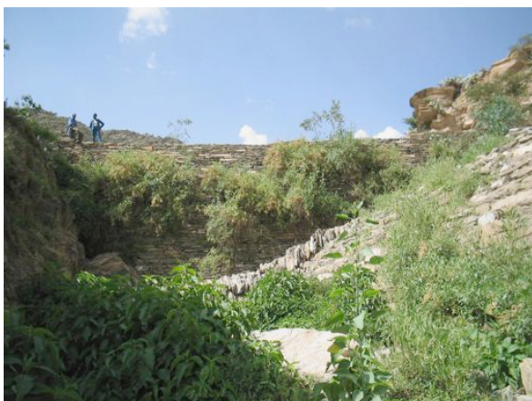
Illustration 7: Topmost check dam of the Dogogola sequence, with soil stabilizing stone embankment at the right side
